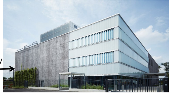
HPC DATA CENTRE PEAK ELECTRICAL LOAD 210 MW
